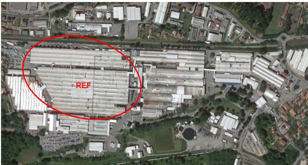
Figure 30: ExFA-IT – Whirlpool's Refrigerators Factory
