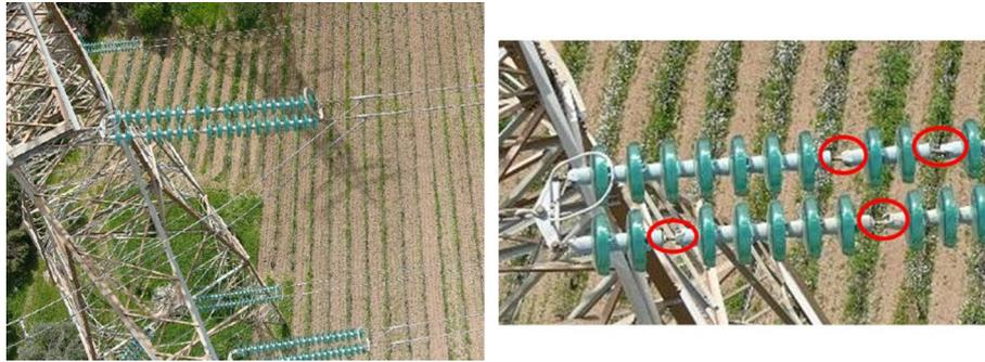
**Fig. 7** Detection of missing insulator stems using federated learning
